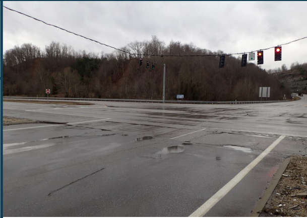
KY 10 looking westbound
