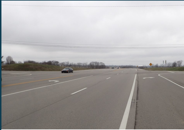
KY 9 looking westbound
