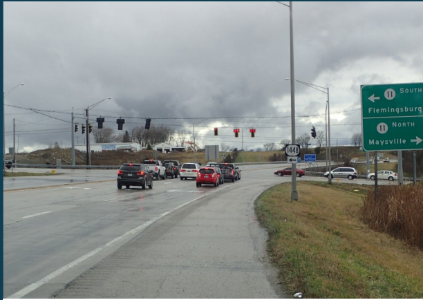
KY 9 looking westbound
