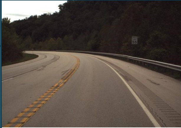
KY 9 looking westbound
