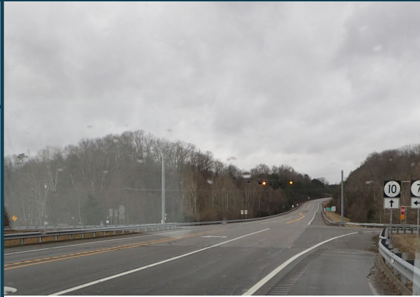
KY 10 looking westbound
