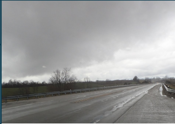
KY 9 looking westbound
