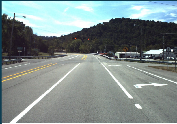
KY 9 looking westbound
