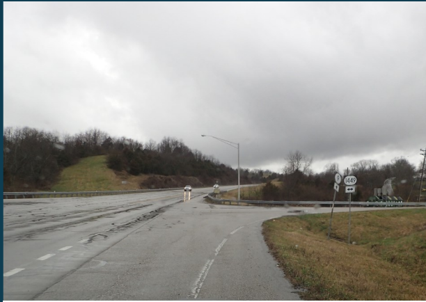
KY 9 looking westbound
