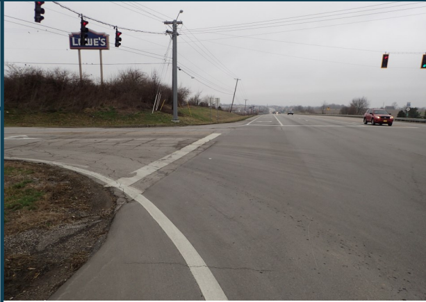
KY 9 looking westbound
