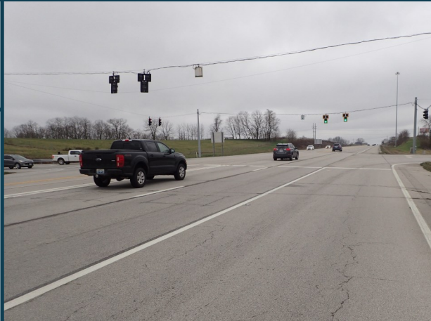
KY 9 looking westbound
