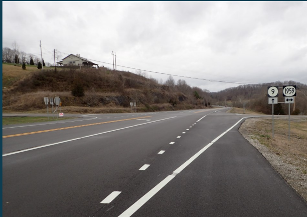
KY 9 looking westbound
