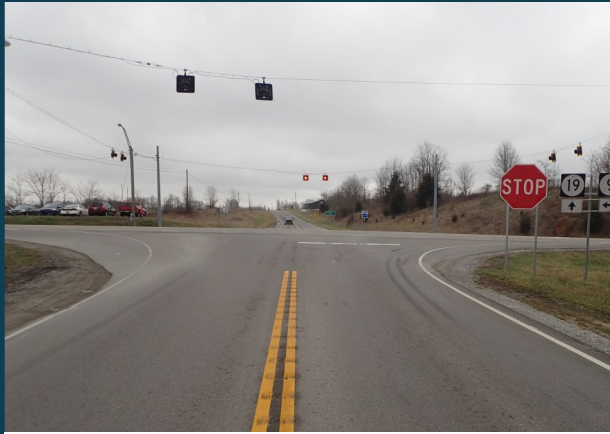
KY 19 looking southbound
