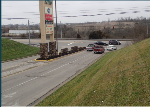
Market Square Drive looking northbound
