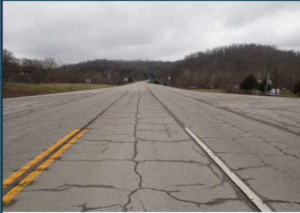
KY 9 looking westbound
