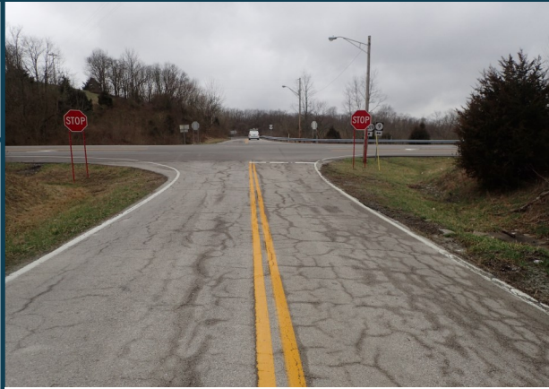
KY 1019 looking westbound
