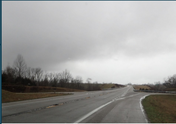
KY 9 looking westbound
