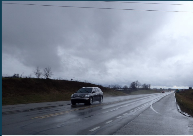
KY 9 looking westbound
