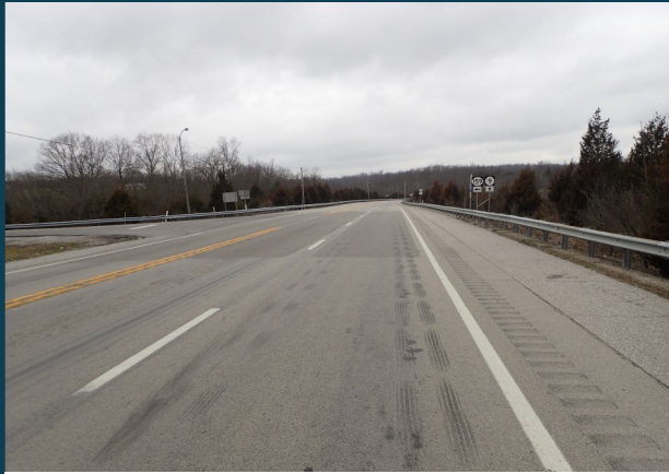
KY 9 looking westbound
