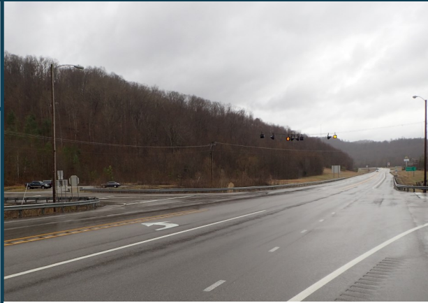
KY 9 looking northbound
