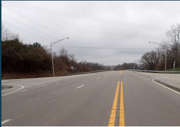
KY 9 looking westbound
